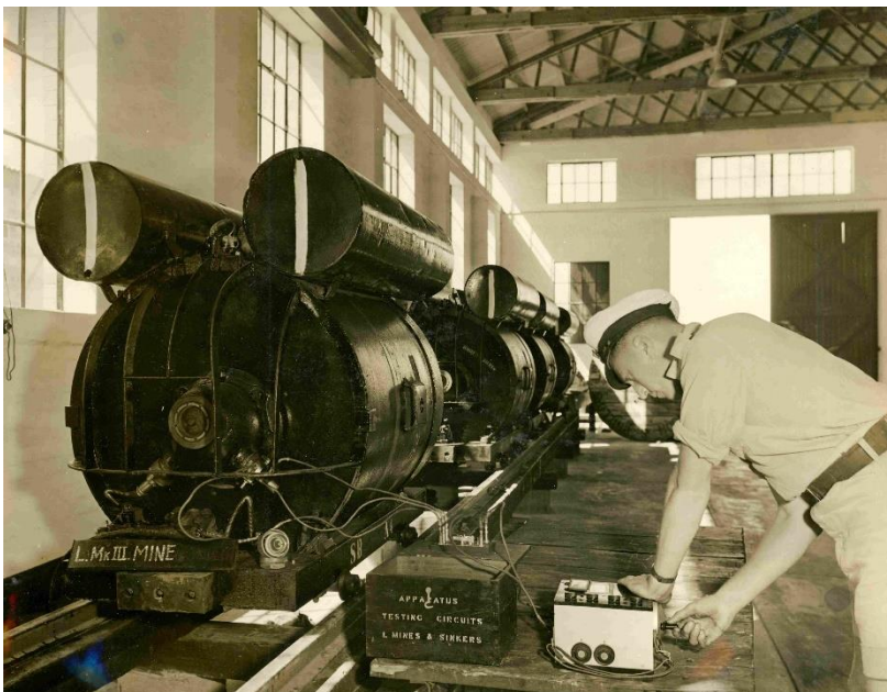
Fig 25: Electrical tests on assembled mines
