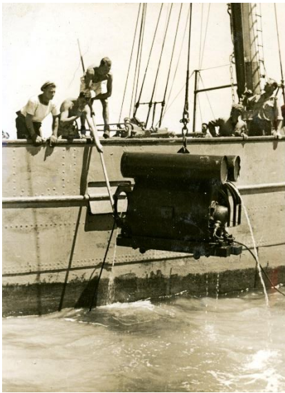
Fig 10: Recovered mine suspended from derrick to allow buoyancy tanks to drain
