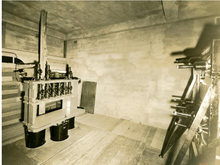
Fig 6: CS84 galvanometer and projector lamps
