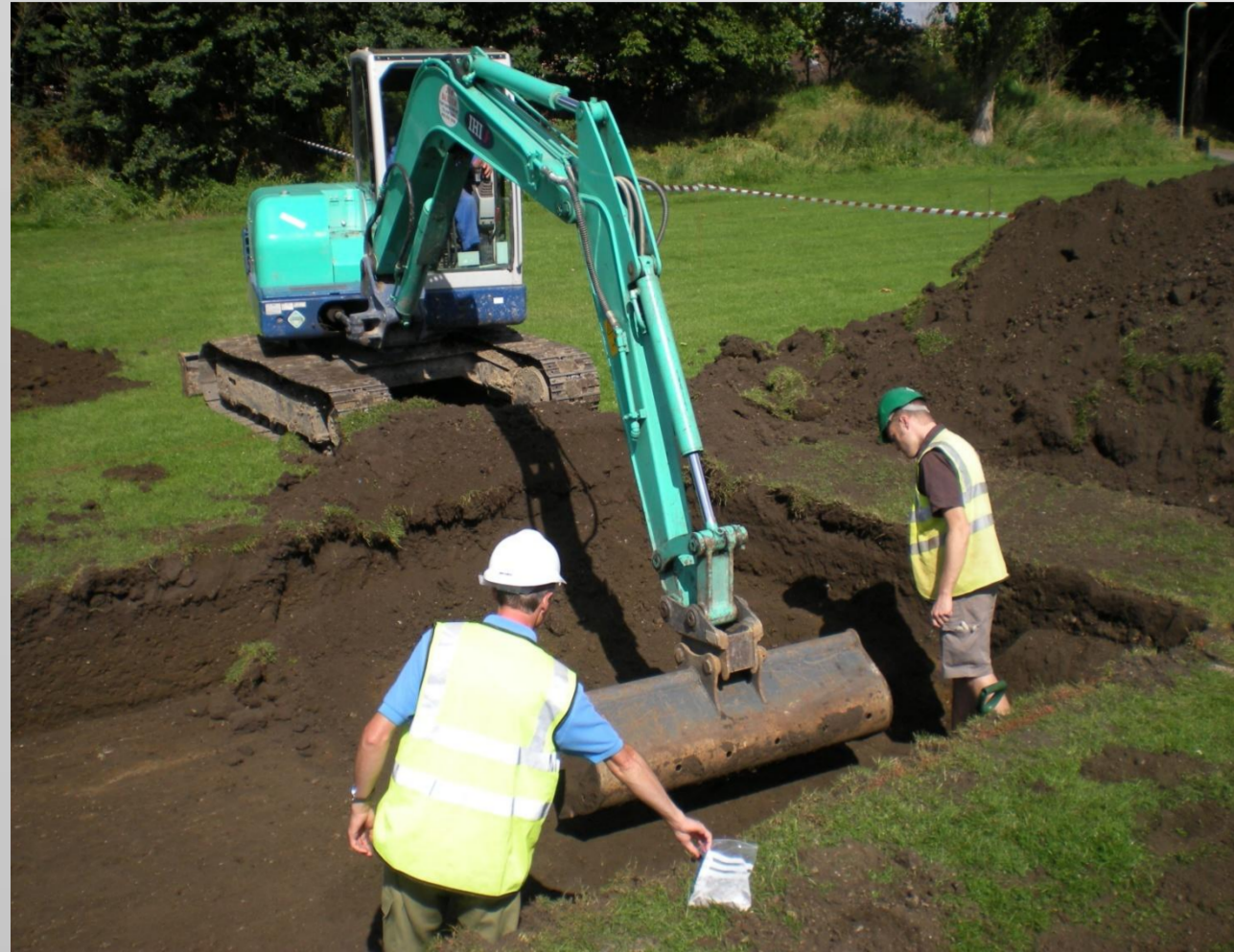
Machining off the topsoil and subsoil layers was performed very carefully, so as not to lose any archaeological deposits
